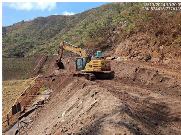
Foto 6.58 – Conexão do acesso principal à berma El. 1.119,0 m.
