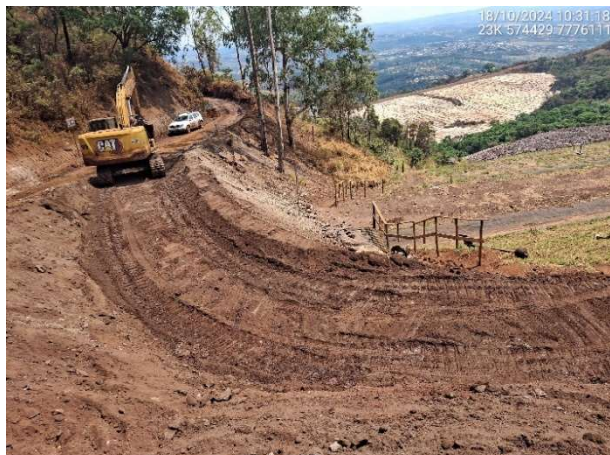
Foto 6.57 – Conexão do acesso principal à berma El. 1.119,0 m.
